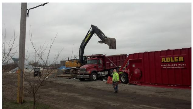
Loading of Tri-Axle Trucks with "A" Group Soil for Offsite Disposal
