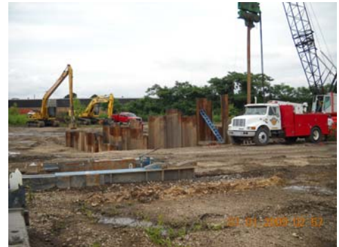
Sheet Piles around the perimeter of excavation area 3
