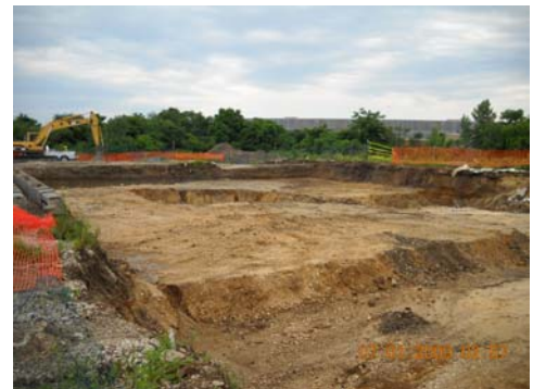
Completed excavation areas 10 and 12
