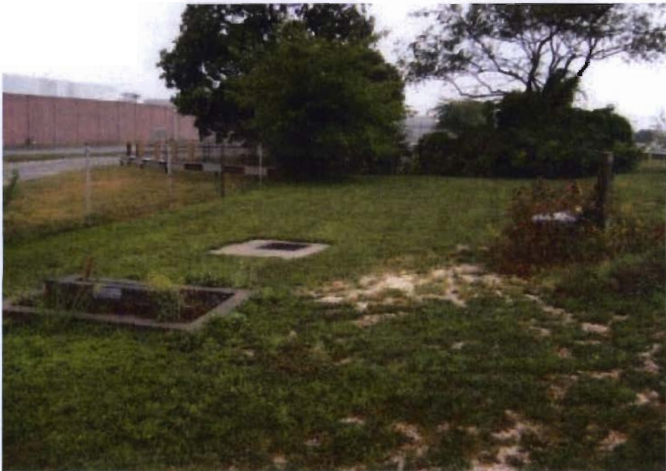
Photo 10 –Site 2, storm water diverter situated in the southeast portion of the Site.
