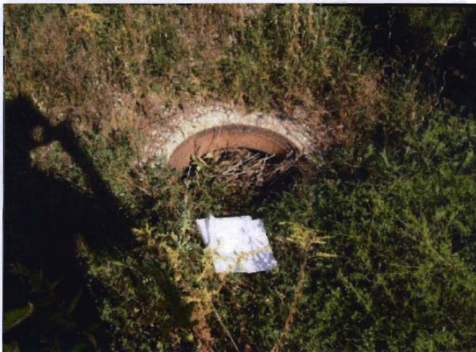
Photo 6 –Site 1, former cesspool.
