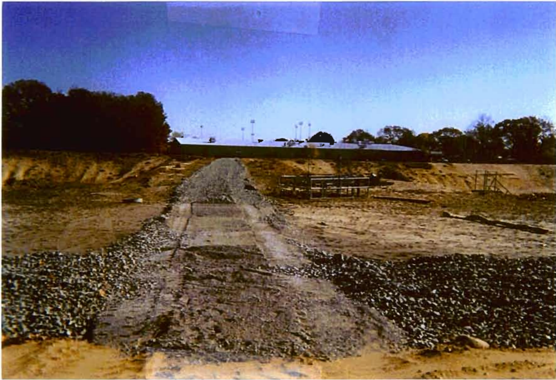
INITIAL CONSTRUCTION OF SITE ACCESS ROAD, LOOKING NORTH
