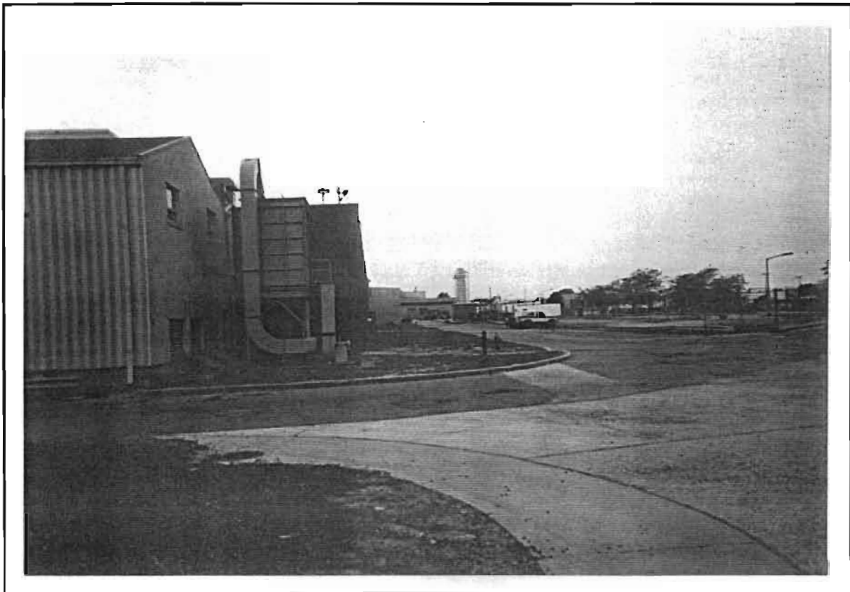
Photo #10 : Northeast corner of plant #3 looking west.
