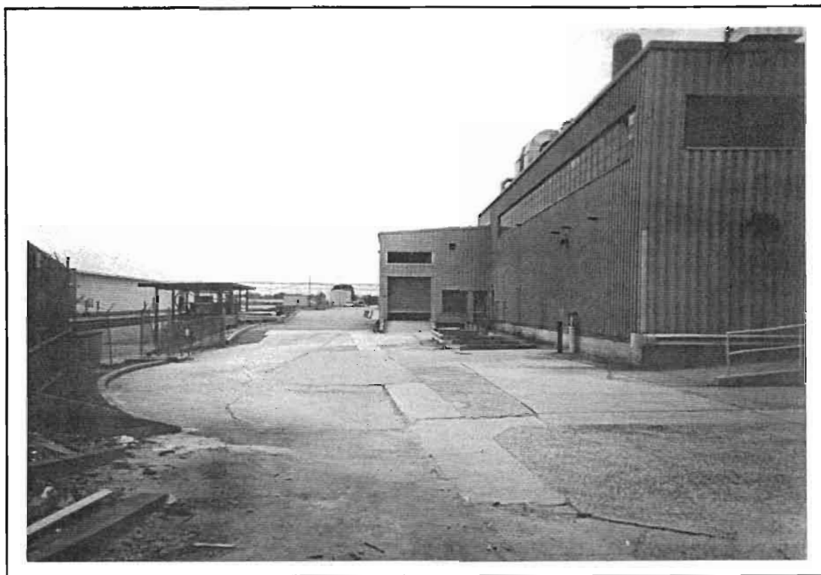
Photo #1 : South side of plant #3 looking west.
