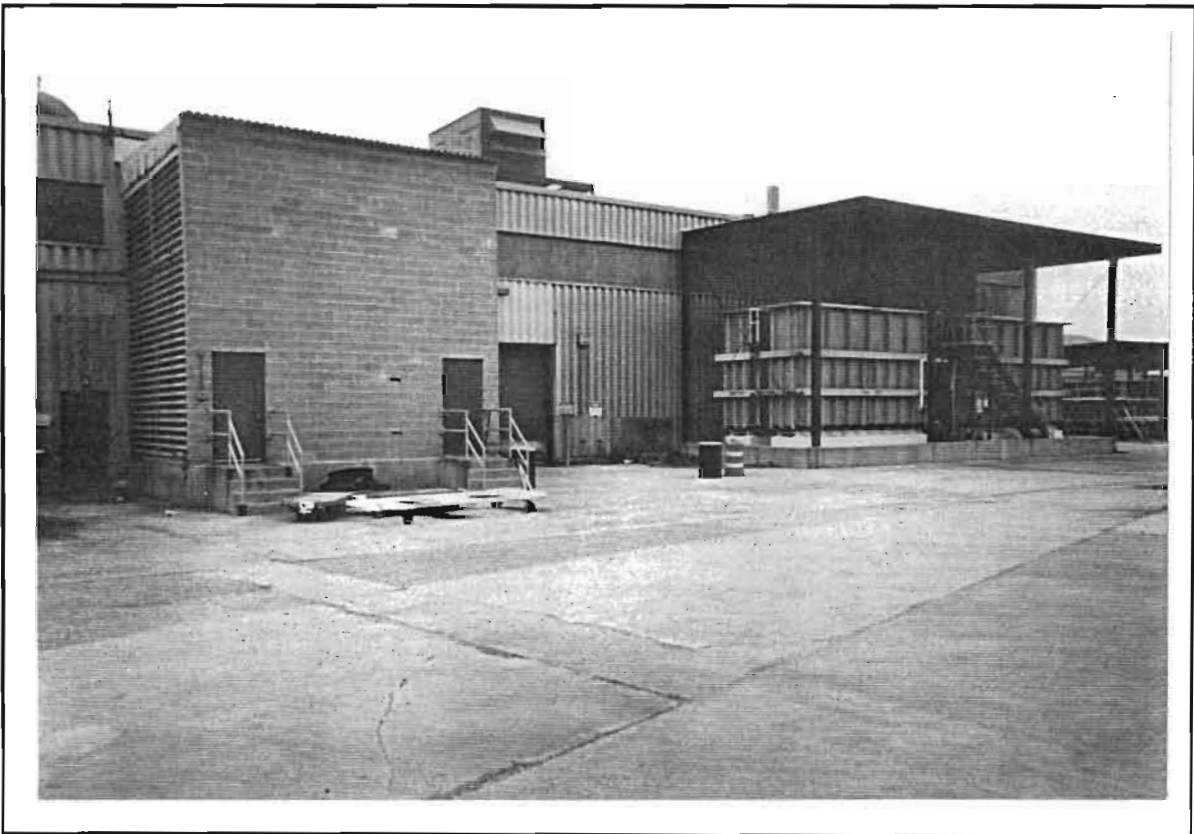
Photo #6 : East side of plant #3 looking northwest.
