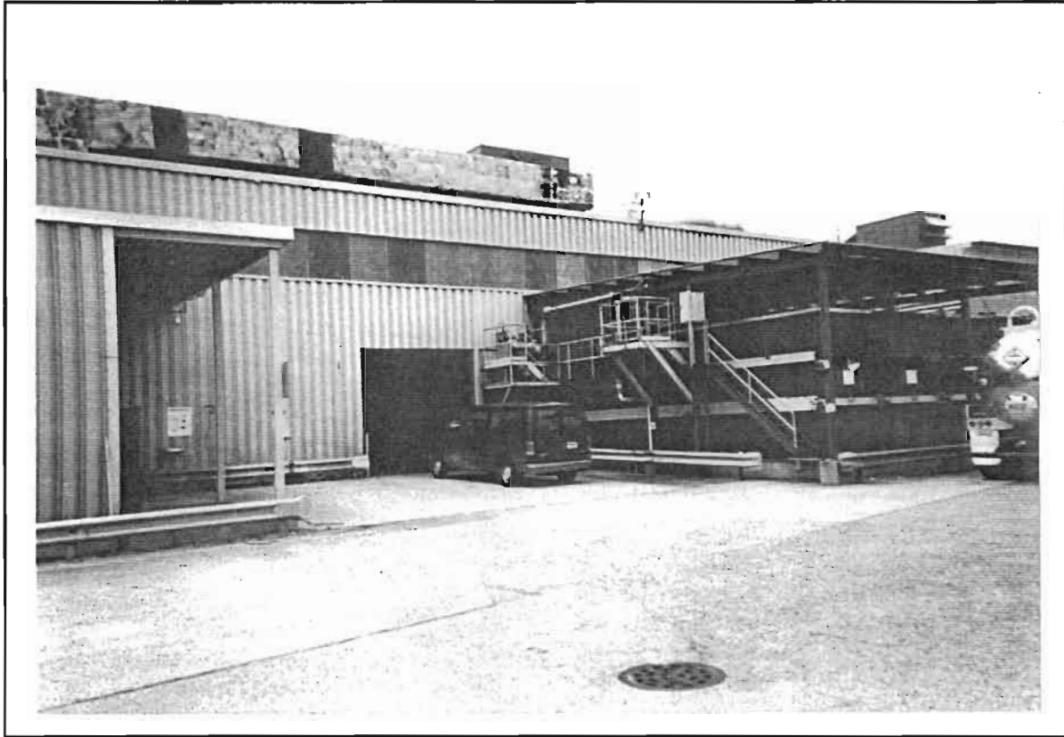
Photo #3: East side of Plant #3 looking northwest.
