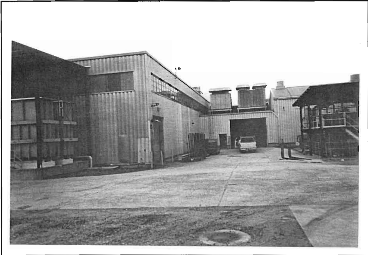
Photo #9 : East side of plant #3 looking west.
