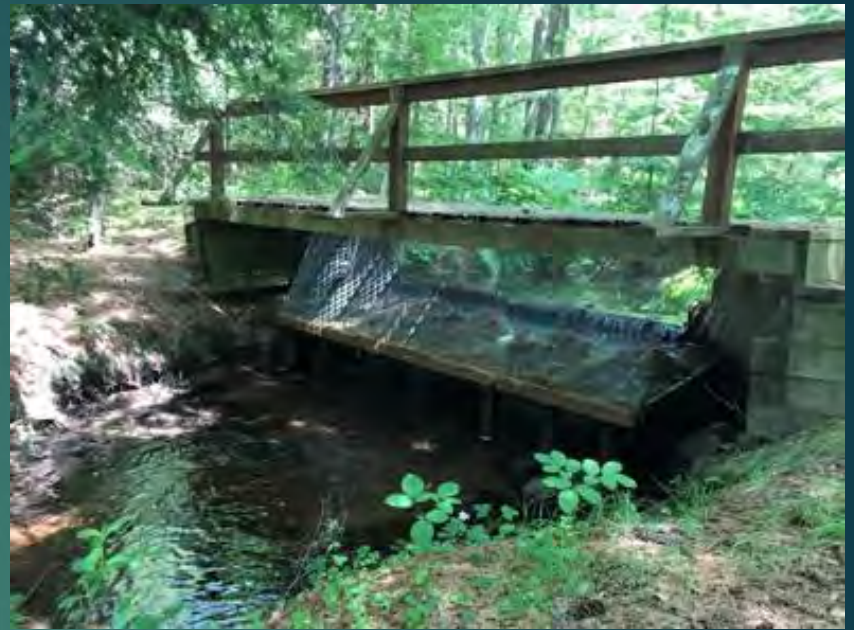
Fish Barrier Dam
