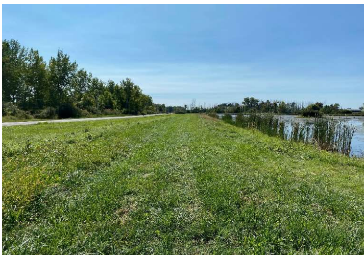
Mud Creek Marsh dike after repairs
