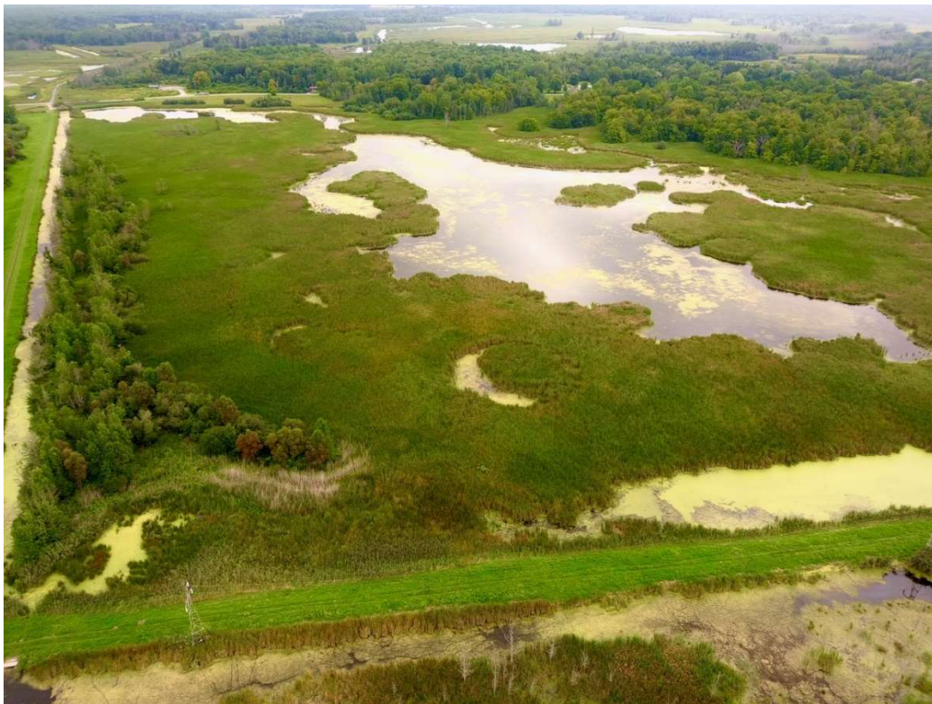
North Feeder (looking north) - late August 2023
