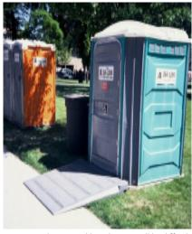
This accessible toilet unit will be difficult for many people with mobility disabilities to enter because they must open the door while on the slope of the ramp. A level landing should be provided.
