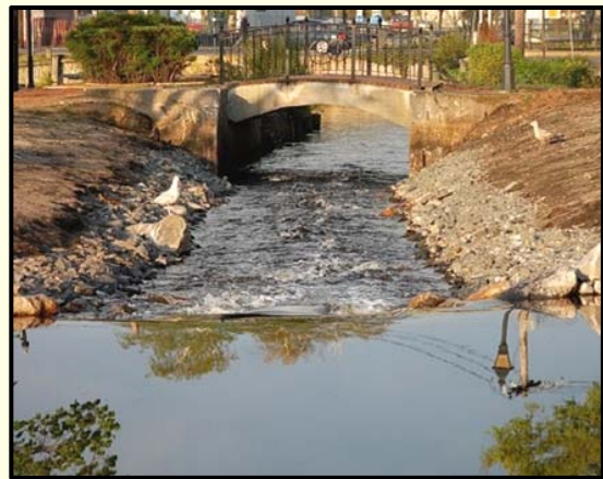
Image: The finished rock ramp fishway at Grangebél Park.
