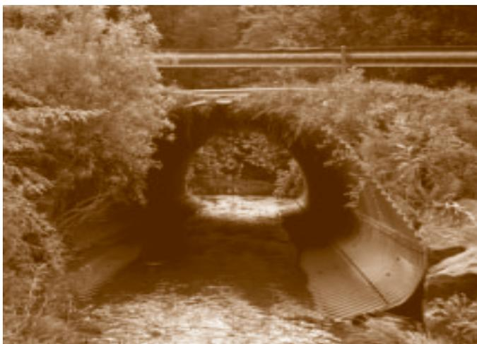
Figure 4. A pipe-arch culvert. These structures may be less prone than round culverts to being plugged by beavers, most likely because they maintain the natural stream width. Additionally, pipe-arch culverts are generally large culverts.
