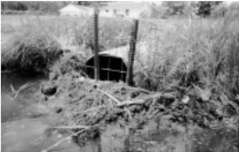
Figure 1. Plugged culvert pipe. Beavers typically use mud, sticks, and other debris to plug culverts. Culvert plugging activity is usually highest during the spring and fall.
