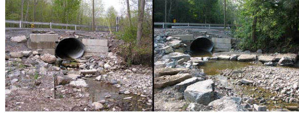
Culvert before and after habitat enhancement work.
