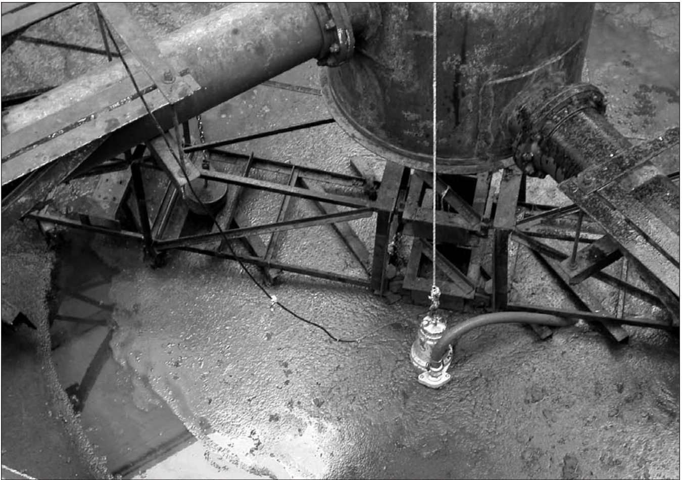
All tanks should be inspected once per year.
