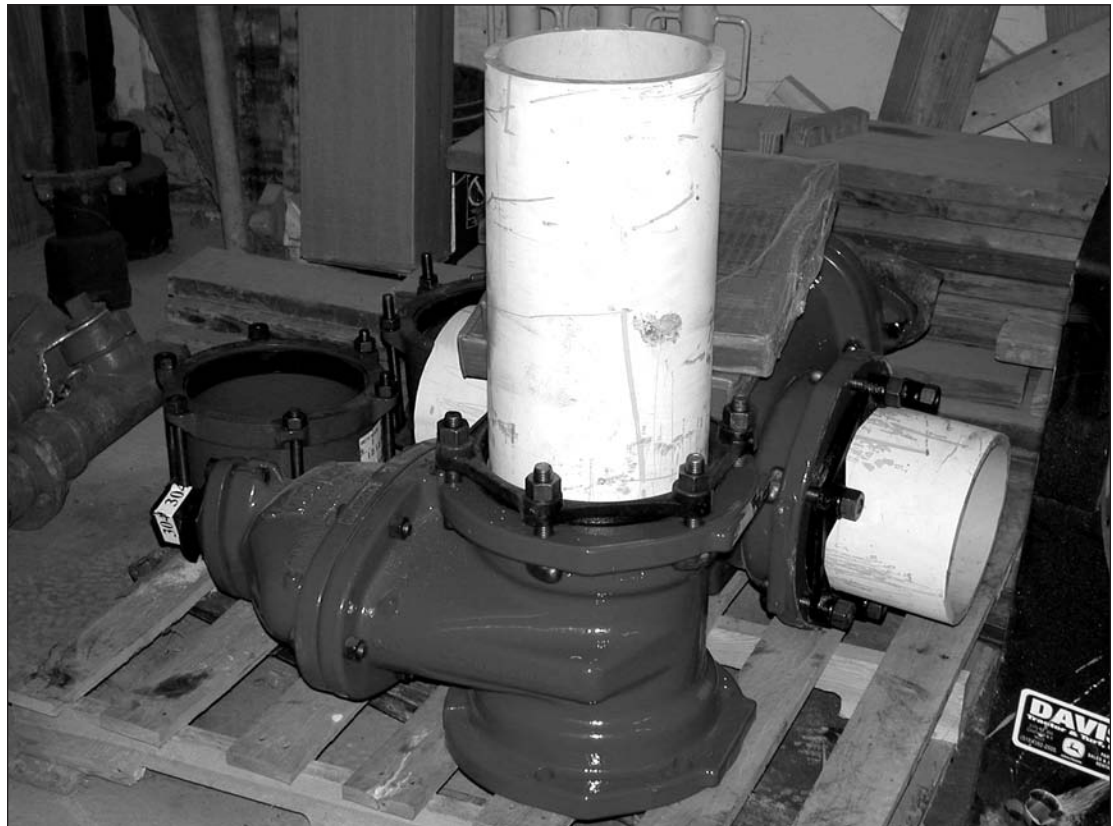
Replacement valve with preassembly awaiting installation
