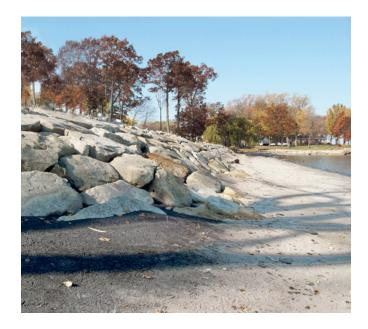
In addition to its recreational and aesthetic features, the presence of a beach waterward of an armor stone revetment will aid in erosion protection.
