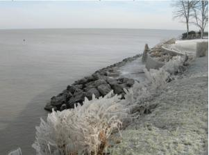
The material should be resistant to erosion caused by run-up and water washing through the armor stone. Fine grained material or a mix of larger material with fines should not be specified.
