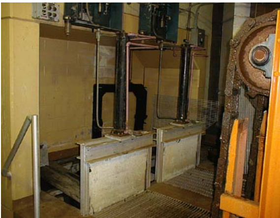
Gate G2 (right) to south bar screen and Gate G3 (left) to North Bar Screen.
