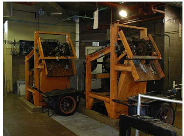
South Bar Screen (right) used for dry weather flow. North Bar Screen (left) ready mode for wet weather event.
