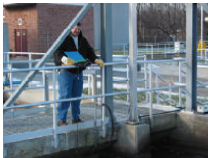
Operator Jack Diagostino measures MLSS in the aeration tank
