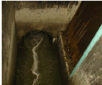
Influent channel with very little storm flow storage before bypass
