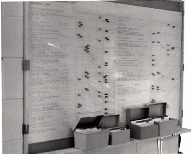
Photo of a wall chart and card system to track maintenance at a smaller wastewater treatment plant.
