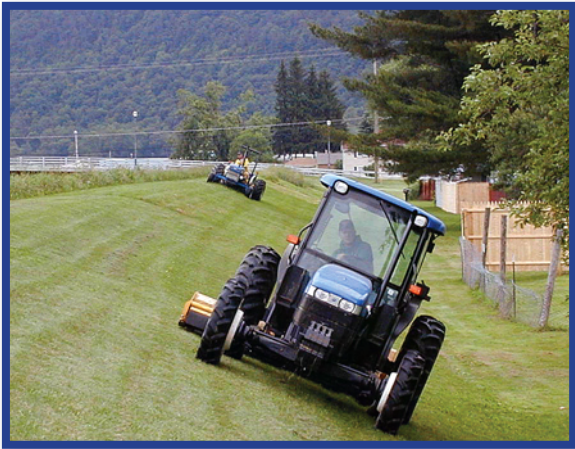
Sod cover protects levees from erosion. Grass length should never be less than four inches.
