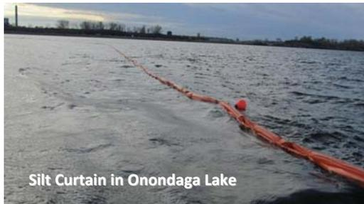
**Navigation Protection** – Measures will be implemented to minimize potential risks to recreational boaters during on-water remediation activities. Navigation protection measures include vessel coordination, lights, marker buoys, and use of a silt curtain designed to contain suspended solids during dredging. Procedures will also be in place for issuing project-related Notice to Mariners and complying with appropriate federal and state navigation laws.
