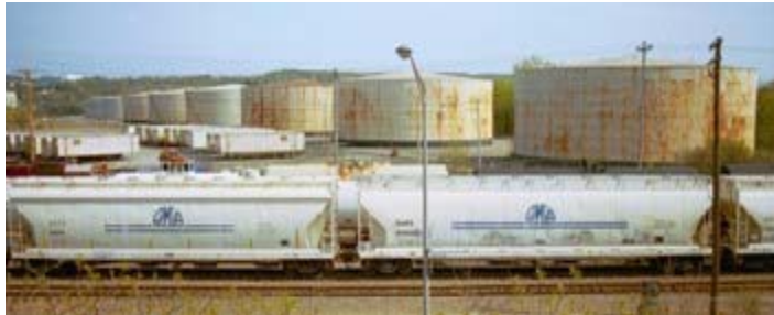
Oil storage facility
