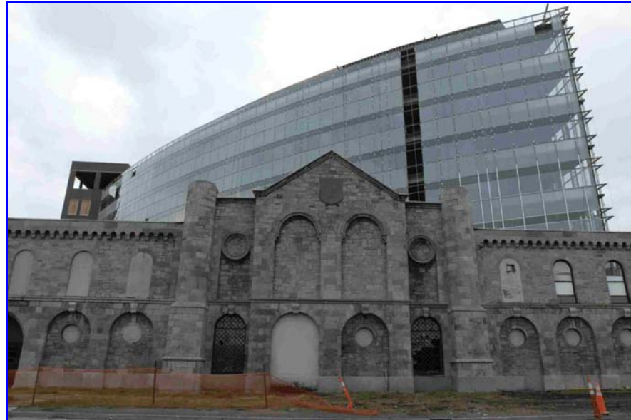
HealthNow, the parent company of Blue Cross/ Blue Shield of Western New York, utilized a Buffalo historic site and brownfield to build its new headquarters.
