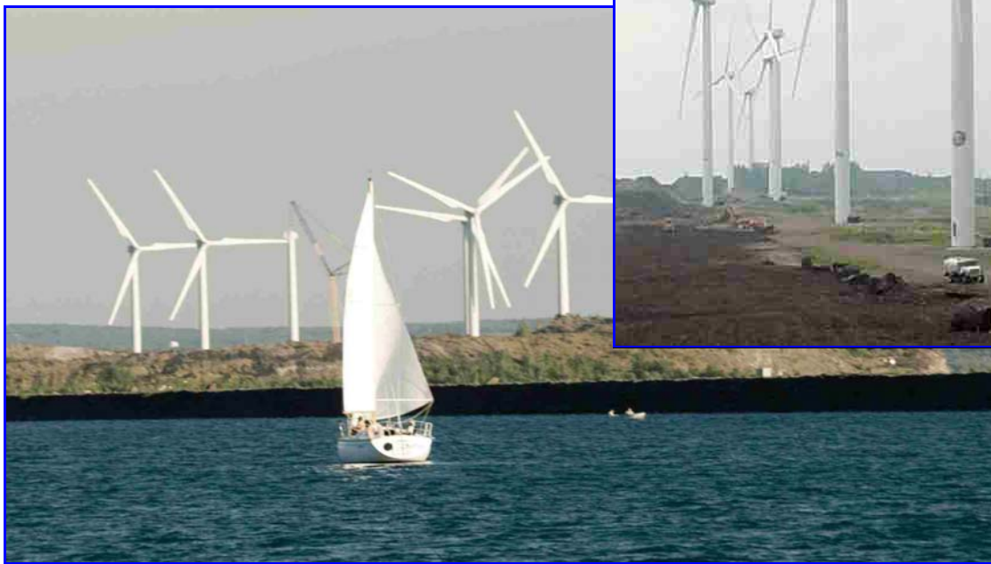
"Winds of Change" - The old Bethlehem Steel site in Lackawanna, is now a wind farm capable of generating enough power for 7,000 homes.
