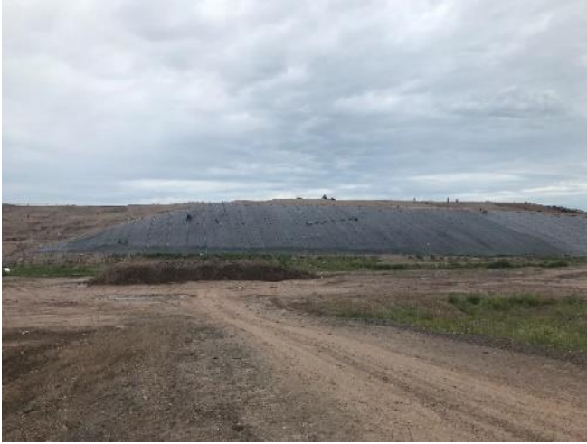
Exposed geomembrane cover over the east side slope of cell 12.
