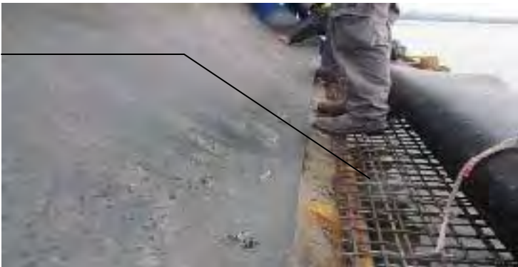
Horizontal Platform with Expanded Metal
