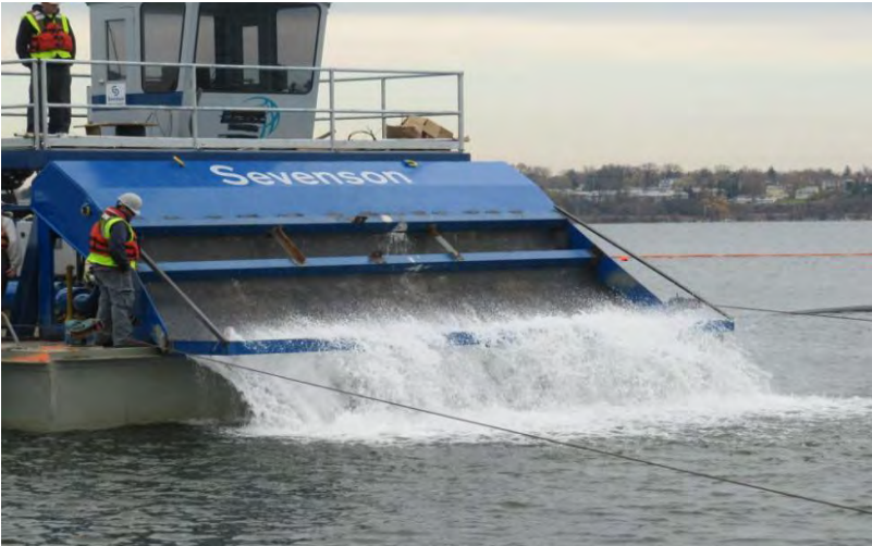
Spreader with Energy Dissipating Belt Addition
