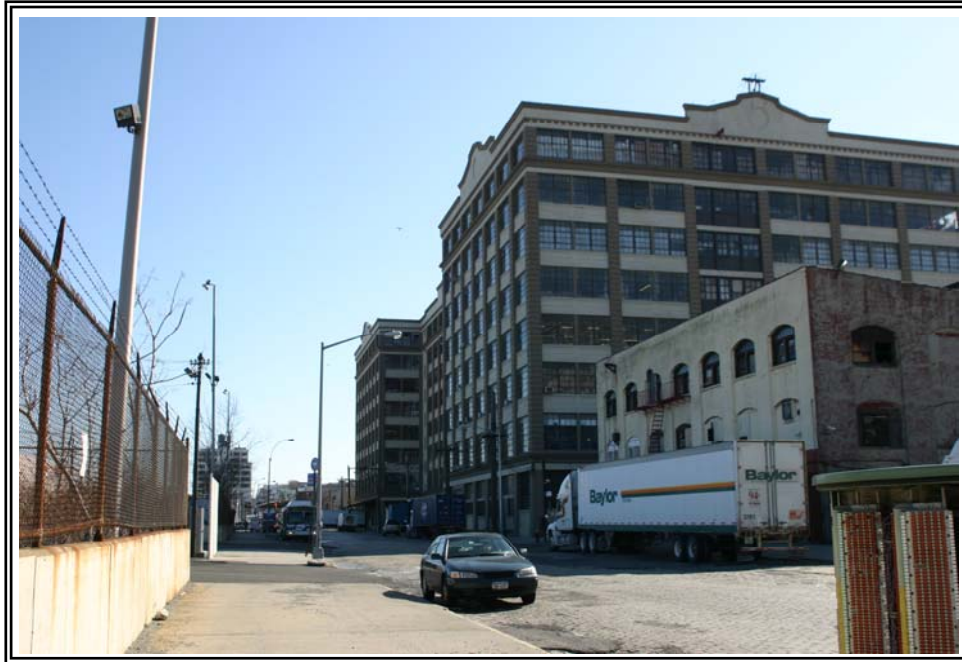
Photograph No. 7, VP-2: Character of Bush complex piers. SPIP is ~0.6 miles to NE
