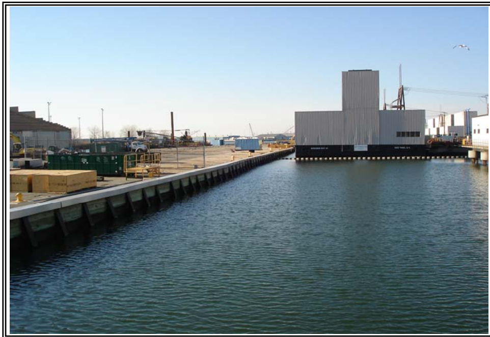
Photograph No. 2: SPIP site to left (south) of GGS barge unit.
