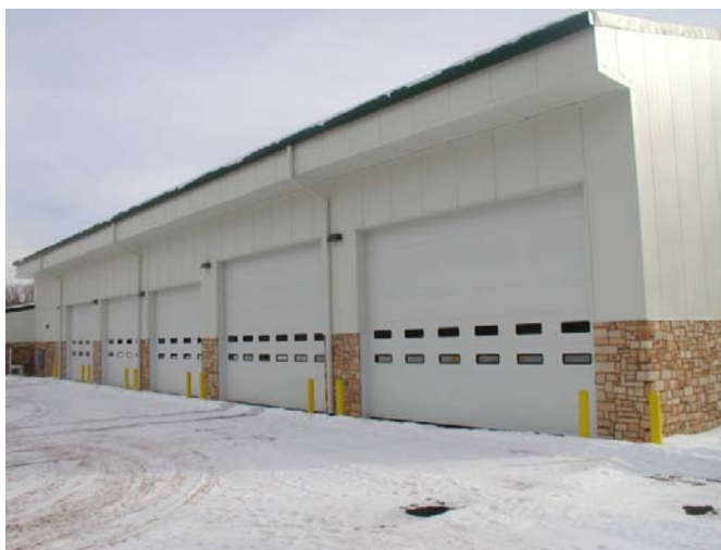
Belleayre Mountain Maintenance Center
