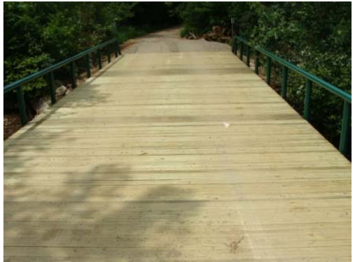
Perkins Clearing Bridge
