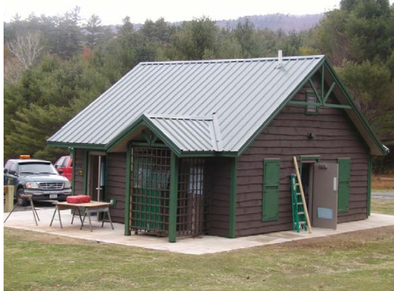
Scaroon Manor Comfort Station & Shower Building
