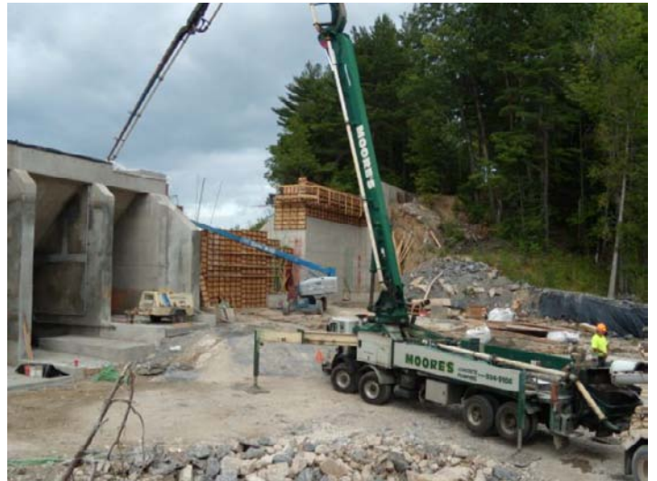
McGregor Dam during Rehabilitation
