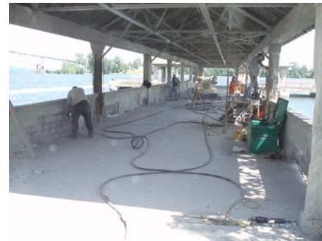
Restoration of Crown Point Pier
