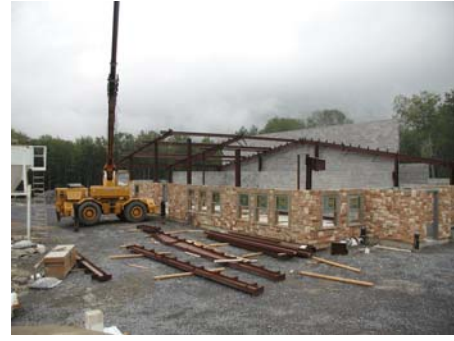
Maintenance Center at Belleayre
