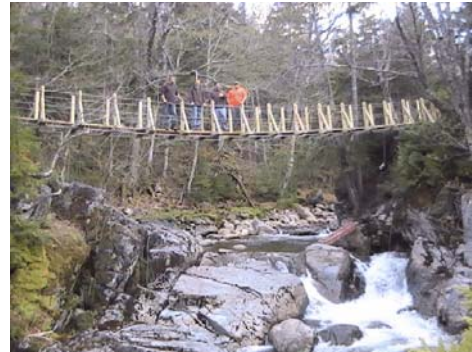
Reconstructed footbridge over Johns Brook
