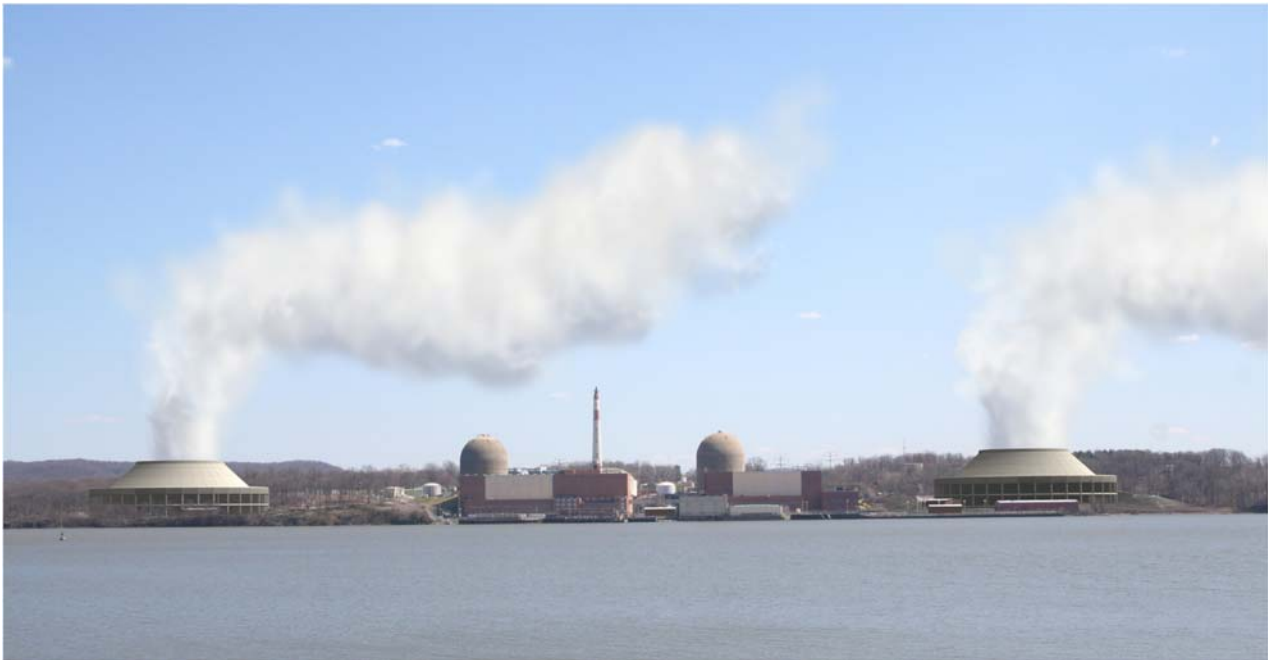
Figure 8.1 Visual Representation of Cooling Towers at IPEC 9
