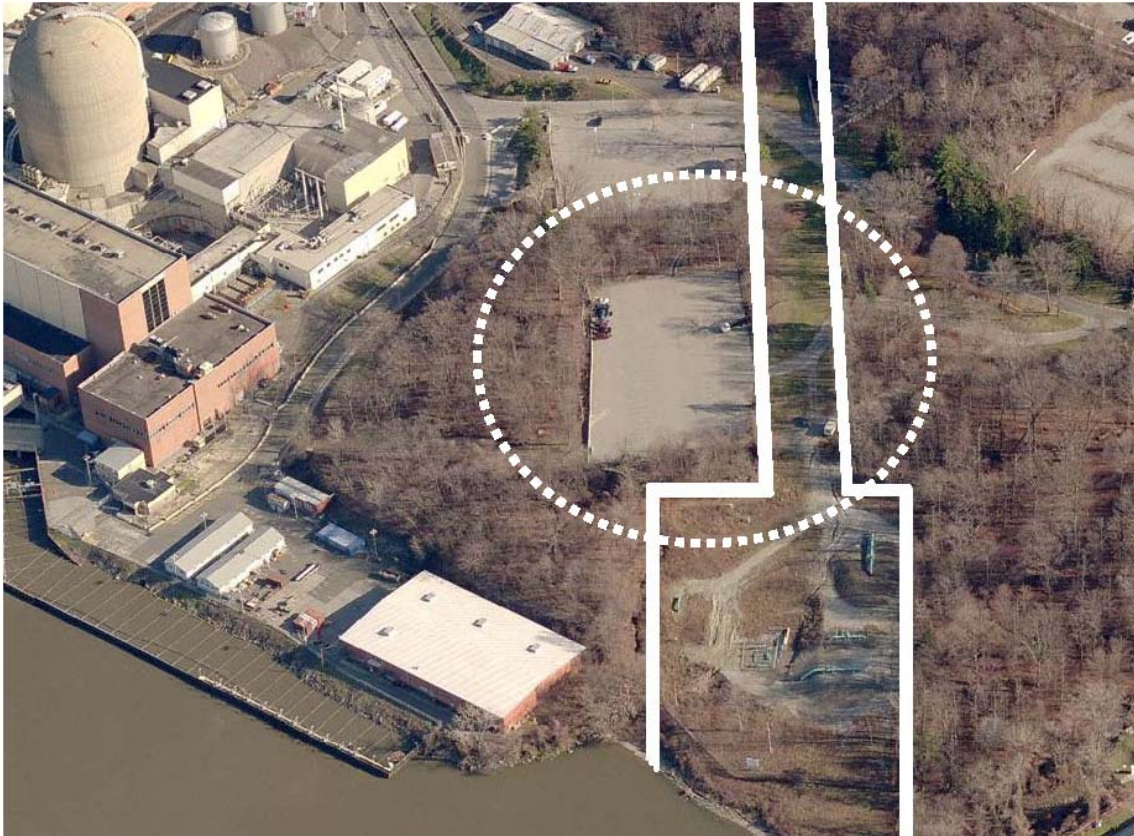
Figure 4.1 Existing Algonquin Gas Transmission Pipeline Right-Of-Way, With Proposed Unit 3 Cooling Tower Location Shown by Dotted Line
