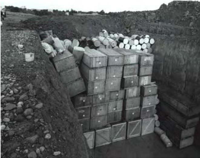
Boxes and drums of radioactive waste stacked in the State-Licensed Disposal Area. Note the water pooled on the trench floor. Photo taken in the mid-1970s.
