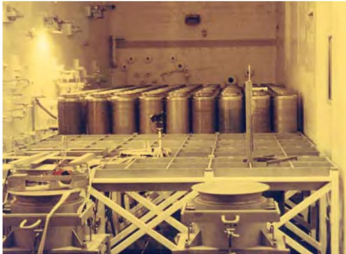
Stainless steel canisters containing vitrified glass logs of high level waste, stored in a "hot cell" room in the Main Process Building.
