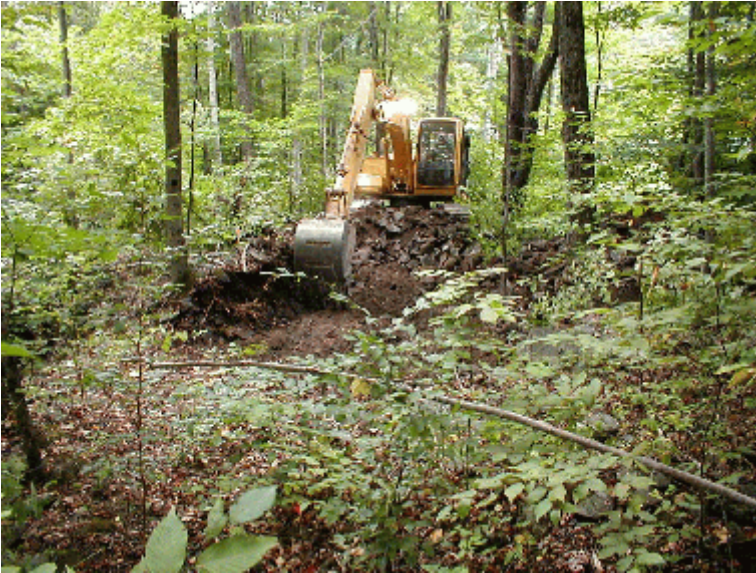
Figure 14 - Horton Brook stream channel restoration project 2001
