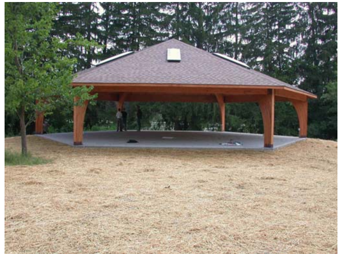
The Finished Outdoor Classroom!
