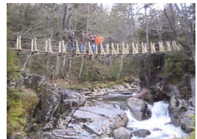
Reconstructed footbridge over Johns Brook
