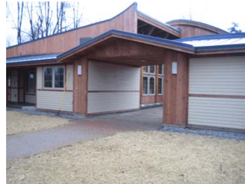
Reinstein Woods Visitor Center is awaiting LEED certification
