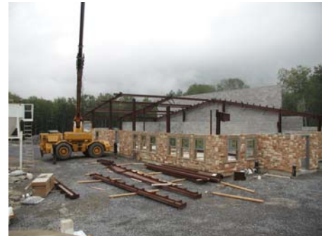
Maintenance Center at Belleayre
