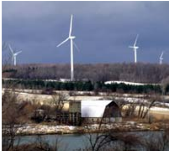
A wind farm with four turbines
