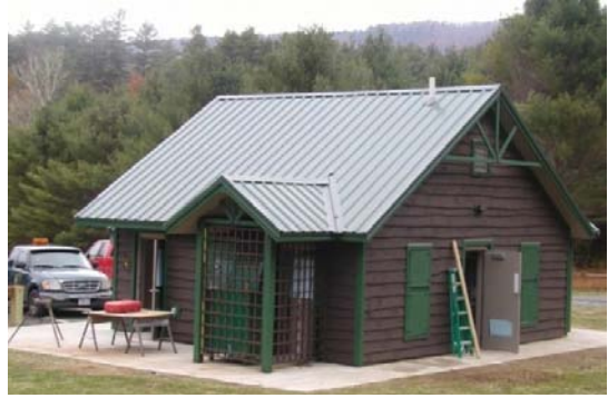
Scaroon Manor Comfort Station & Shower Building
