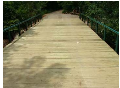
Perkins Clearing Bridge
