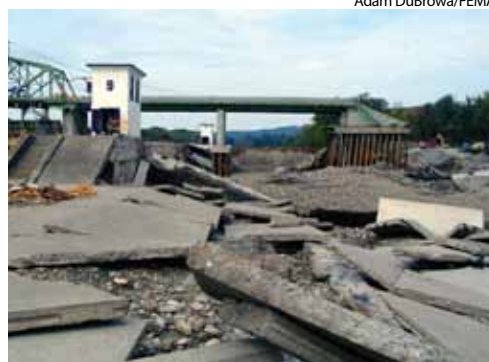
Flooding at Lock 9 of the NYS Barge Canal on the Mohawk River at Rotterdam Junction severely damaged the lock and a nearby bridge.
